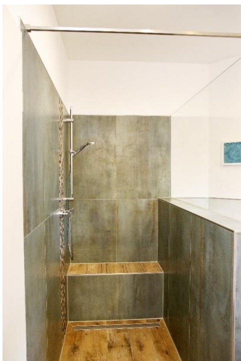
Show house – floor-level shower with seat
