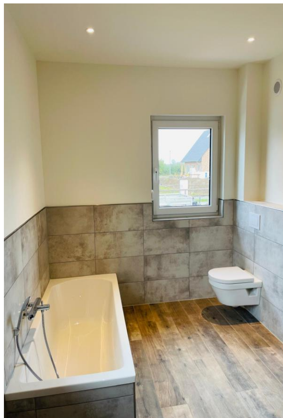
New building – bathtub – toilet
