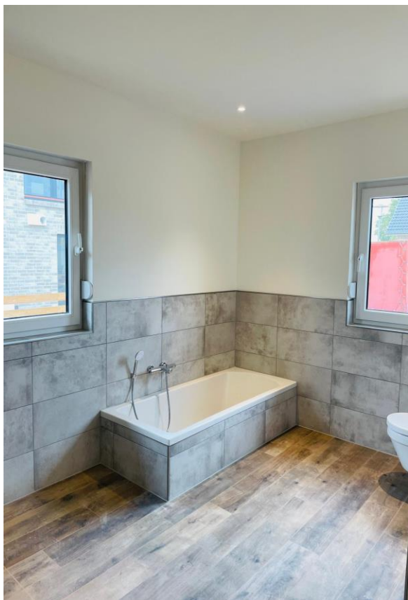
New construction - bathtub
