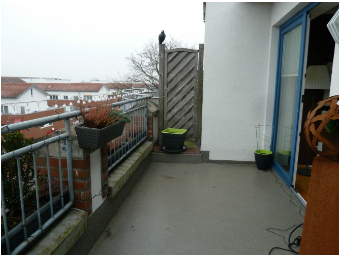
West-Dachterasse (ca. 10 m 2 )
