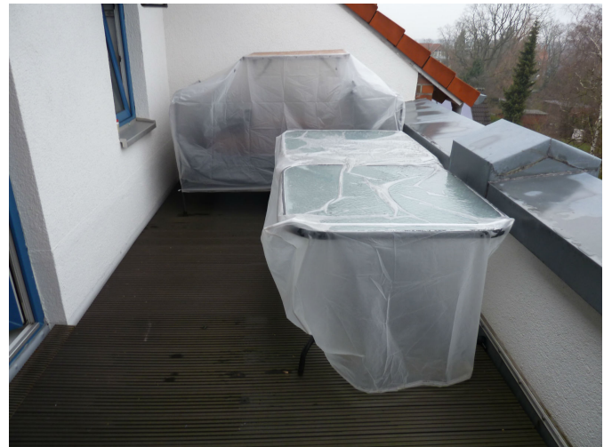
Ost-Dachterasse (ca. 10 m 2 )
