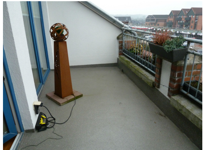
West-Dachterasse (ca. 10 m 2 )
