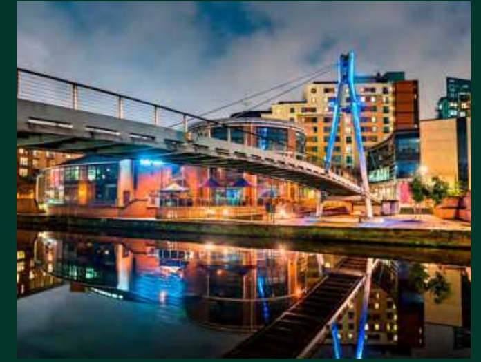
Footbridge across the Aire River
