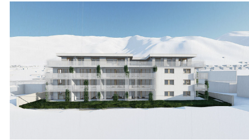
WA STEINA - Steinach am Brenner
